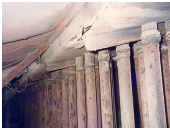
Figure 4: Internal Inspections Identifying Air In-Leakage
