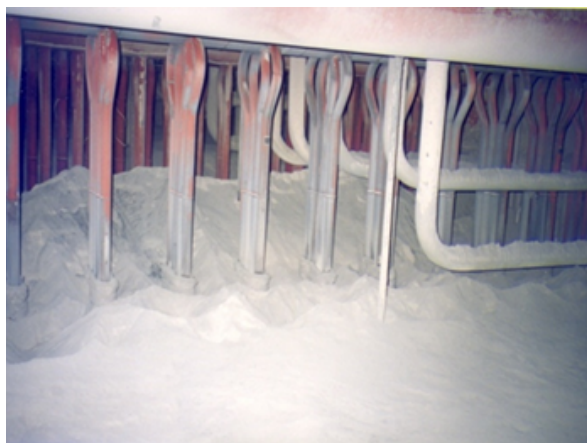
Figure 4: Internal Inspections Identifying Air In-Leakage
