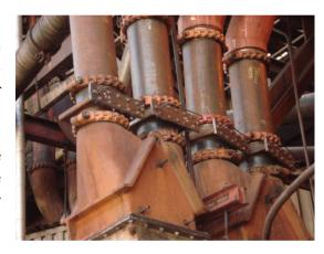
ease of maintenance. We have seen adjustable orifice mechanisms seize during operation and fixed spool OEM orifices no longer being the indicated orifice size opening due to years of wear and regular maintenance neglect. STORM engineers have designed a simplified orifice assembly that houses a 3/8" thick AR400 square-edge orifice plate. Many of our customers prefer this option due to in simplicity, safety, ease of installation and maintenance, and possible fuel line isolation opportunities.
