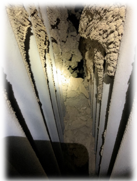
Figure 3: Furnace Slagging Resulting in a Forced Outage
