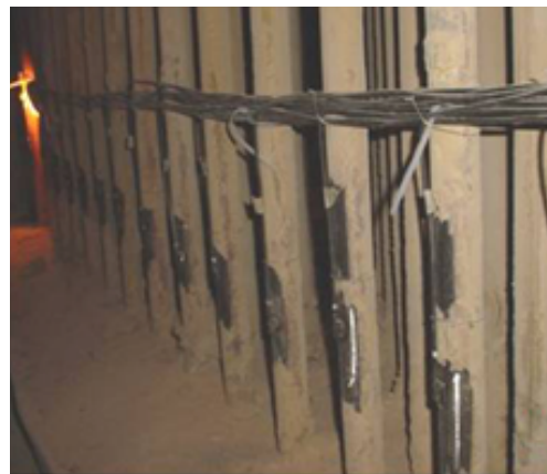
Figure 1: Tube Metal Thermocouples (Left); After Insulation (Right)
