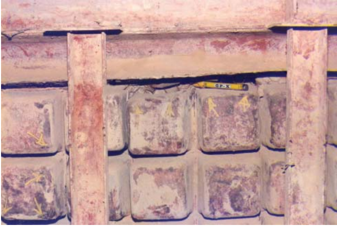
6. From every direction. “Cupcake” expansion joint leaks at the economizer of a 585-MW supercritical boiler show air in-leakage from four sides and numerous cracks/tears. Total leakage was estimated to be equivalent to 5% of total combustion air. Courtesy: Storm Technologies Inc.
