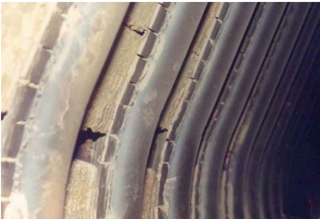
8. Penthouse ash accumulation accompanies air leakage. The before photo (top) shows buildup of ash; the after photo (bottom) shows the same area after repairs were begun. Courtesy: Storm Technologies Inc.
