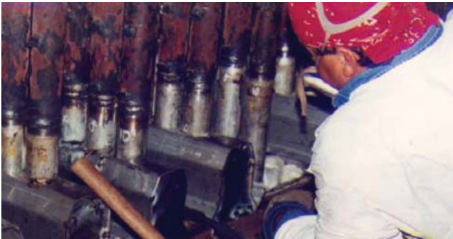
8. Penthouse ash accumulation accompanies air leakage. The before photo (top) shows buildup of ash; the after photo (bottom) shows the same area after repairs were begun. Courtesy: Storm Technologies Inc.
