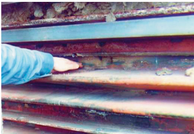
Figure 2. Massive air in leakage path made possible by the coal ash erosion of the thin metal expansion joint at the economiser outlet flue gas location, upstream of the boiler oxygen analysers.
