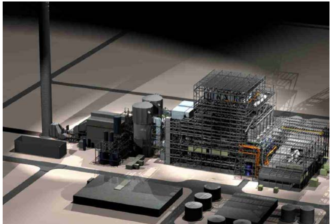
Architect's rendering of AEP's John W Turk Jr Plant, the first ultra-supercritical generating unit.
