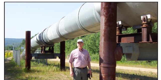
This is the 48" Alaska Pipeline. About one million barrels of oil flow through this daily. America uses about 21 million barrels of oil per day, so imagine 21 of these 48" pipes lined up side by side. This is what powers American transportation on the roads, in the air and over the rails.
