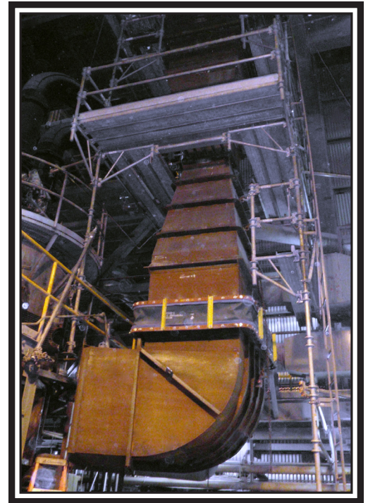
Actual Duct Being Installed
