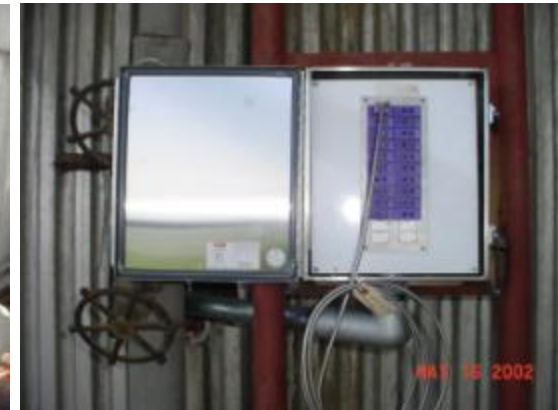
Primary Super-Heat (PSH) Element Tube Metal Thermocouple Installation Progress
