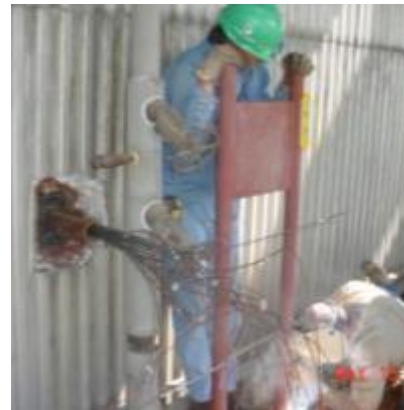
Primary Super-Heat (PSH) Element Tube Metal Thermocouple Installation Progress
