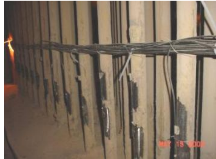
Installation of PSH Tube Metal Thermocouples
