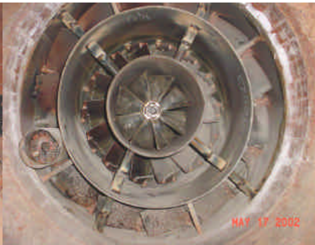
Figure 15 Burner after repairs
