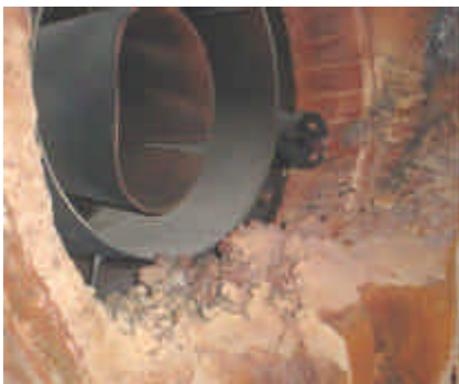
Figure 30: "As Found" Burner Tolerances
