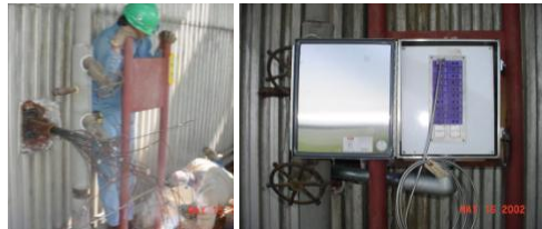
Primary Super-Heat (PSH) Element Tube Metal Thermocouple Installation Progress
