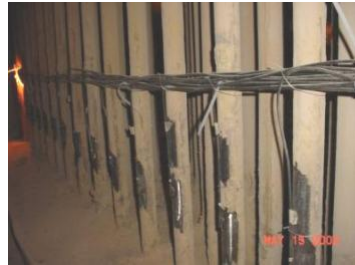
Installation of PSH Tube Metal Thermocouples
