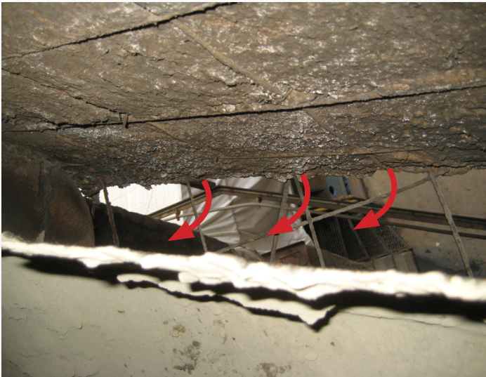
Above: ID fan inlet housing hole (major source of air in-leakage)
