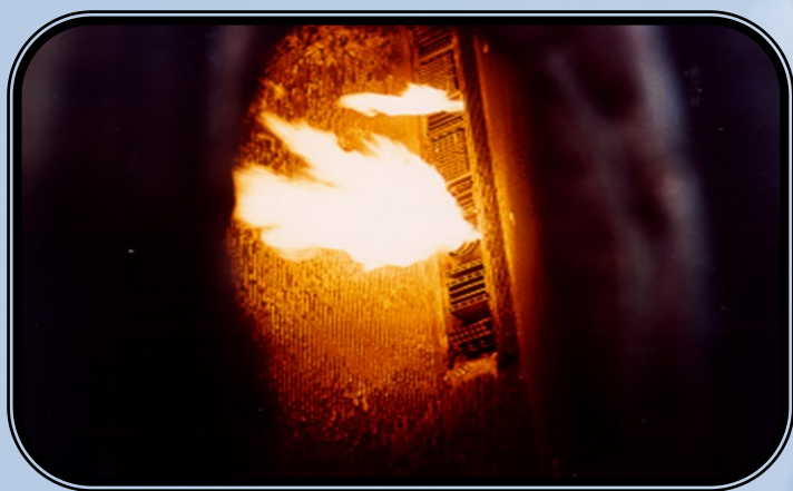
Figure 5. Flame observed after 1–2 auxiliary compartment opened to provide more combustion air. This resulted in less than 10% opacity.
