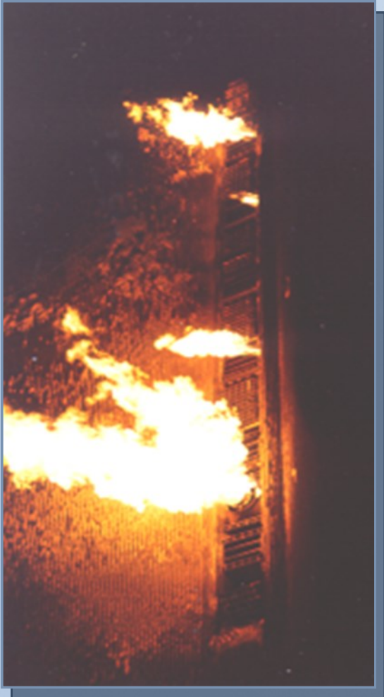
Figure 2. Warm up guns and ignitors with insufficient air for complete combustion; approximately 40% stack opacity.
