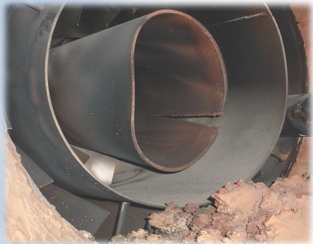
Figure 3. Heat damaged burner nozzle
