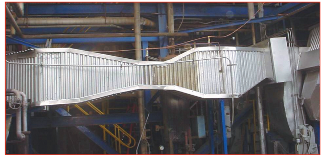
Figure 10. Flow nozzles.
